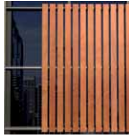
INSTALLATION OF PROFILES FOR VERTICAL LOUVERS
