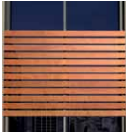
INSTALLATION OF PROFILES FOR HORIZONTAL LOUVERS
